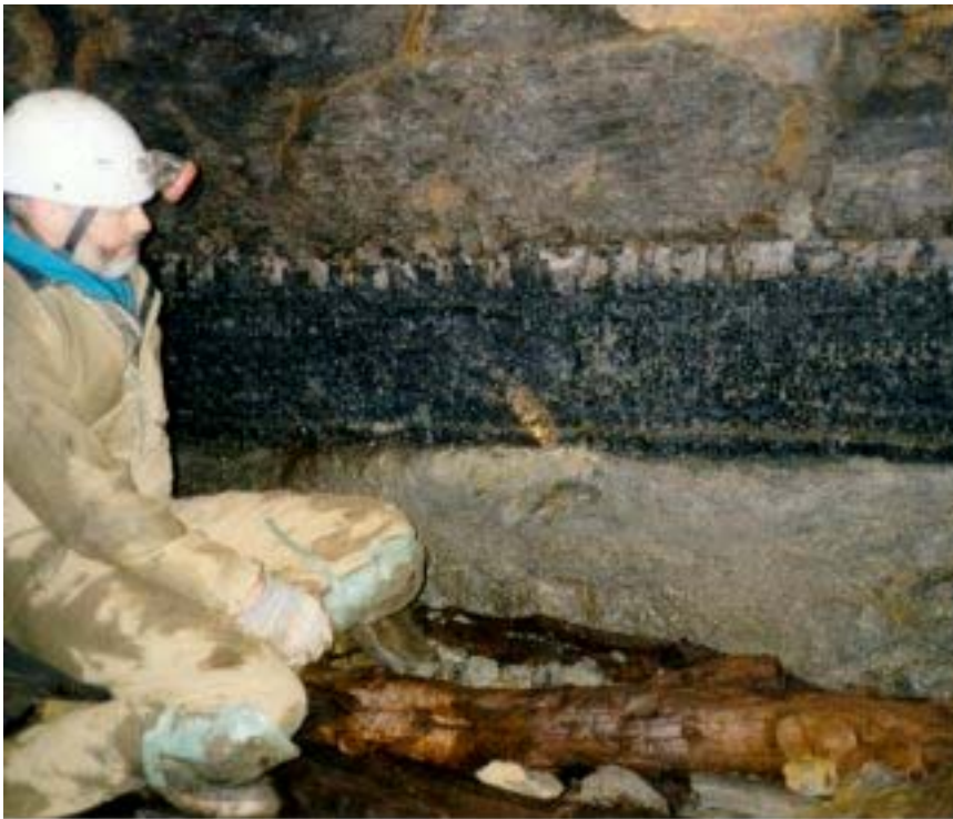
The layer of grey fireclay can be clearly seen below the coal seam. This picture was taken under the summit of Winter Hill fairly close to the moorland road leading to the TV mast. This tunnel is now not accessible and this may be the last picture you ever see of it.
